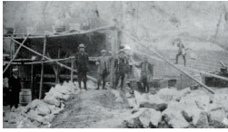
Railway laying project for Seiso Electric Railway
