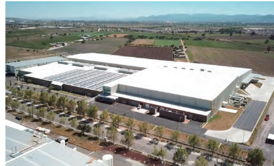
Mitsubishi Electric Querétaro Factory [Mexico, 2020] → Details https://www.fujita.co.jp/works/317/
