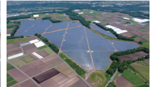
Solar power equipment in Hitachi Showa Village
