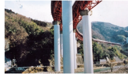
Reinforcement of Sakawa River bridge, Tomei Expressway
