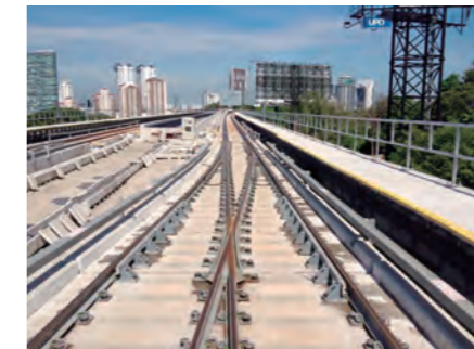
Malaysia KVMRT NO.1 Line Slab Track Construction [Malaysia, 2016] → Details https://www.fujita.co.jp/works/1736/
