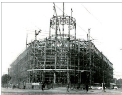
Metropolitan Police Department steel frame project
