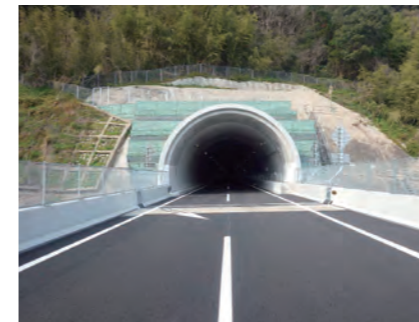
Nakao Tunnel, Nagasaki Expressway [Nagasaki, 2019] → Details https://www.fujita.co.jp/works/601/
