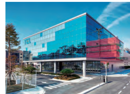
Tokyo Electron Korea Ltd. PTSC (Pyeongtaek Technical Support Center) [South Korea, 2019] → Details https://www.fujita.co.jp/works/453/
