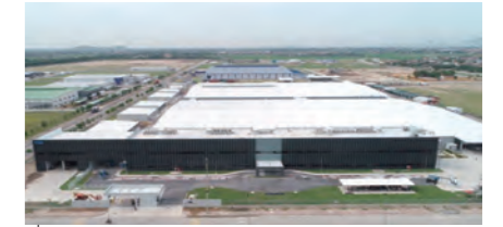
Factory in Hanoi for YKK Vietnam [Vietnam, 2019] → Details https://www.fujita.co.jp/works/474/
