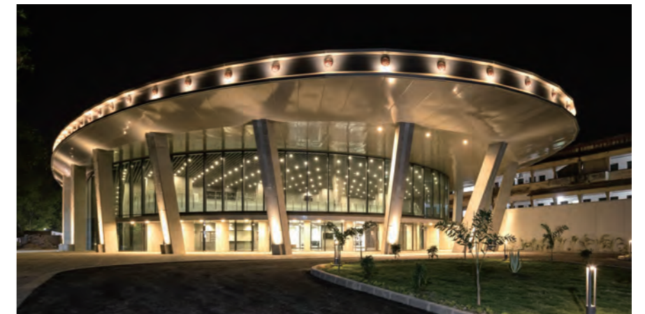
RUDRAKSH - International Cooperation and Convention Centre [India, 2020] → Details https://www.fujita.co.jp/works/4329/
