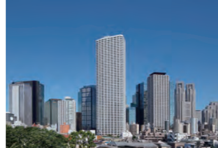
Urban renewal in center-north of Nishi-Shinjuku 5-chome [Tokyo, 2017] → Details https://www.fujita.co.jp/works/1746/
